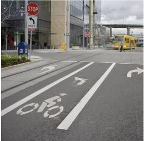
Left turn bike pocket to encourage track crossing at a safer angle at Bond and Whitaker in Portland.
