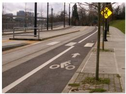
Center-running track with center platform in Portland on SW Harrison: The center platform eliminates the pinch point at curb extension platforms, while the lack of parked cars eliminates conflict with parking cars and doors.
