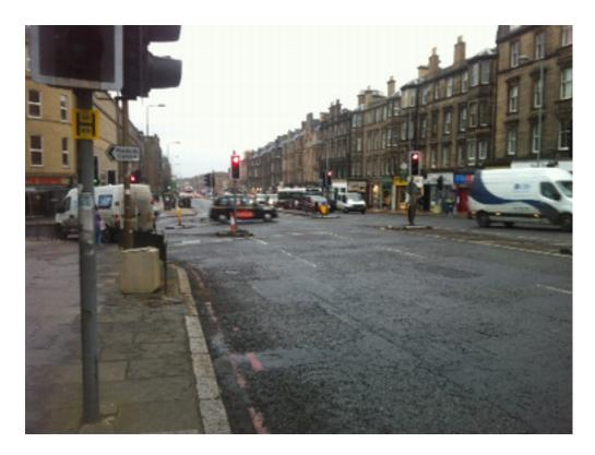
The left-turn feeder lane for northbound traffic turning into Annandale Street, and the central traffic islands, should be removed, with only two traffic lanes approaching the junction. Also, the angle of the turning into Annandale Street should be sharpened by pavement widening, so that the whole junction becomes smaller scale and more appropriate to an urban shopping street.
