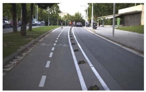
Example of a semi segregated cycle lane (Picture courtesy of Transport for London) in which armadillos are placed between mandatory cycle lane markings. In the case of Meadow Place Road the cycle lane would be unidirectional.
