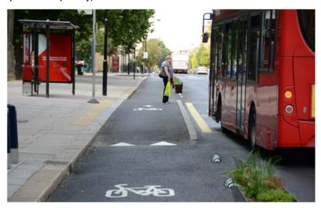
Example of bus boarding / cycle lane arrangement (Picture courtesy of Alex Sully)
