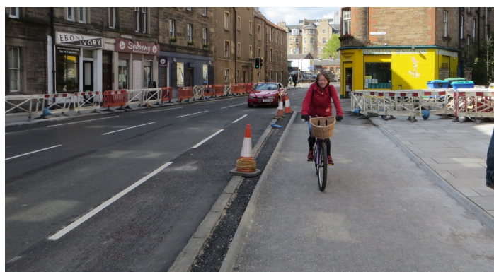
Edinburgh's first segregated onstreet lane under construction, a link in the Meadows-Innocent route photo DdF
