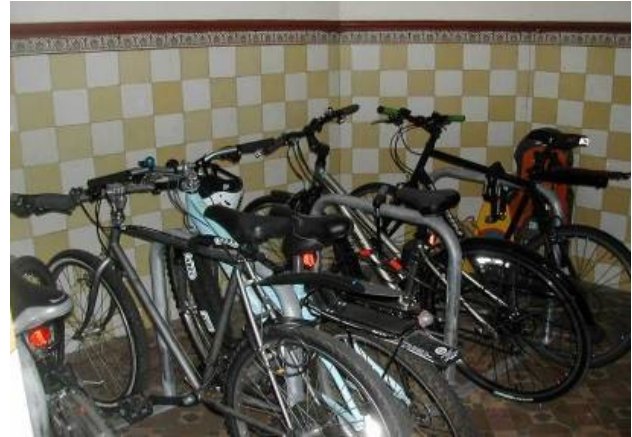
Stairwell Toast-rack - Sheffield stands welded to a base frame which rests on the floor [Sam Anwar]
