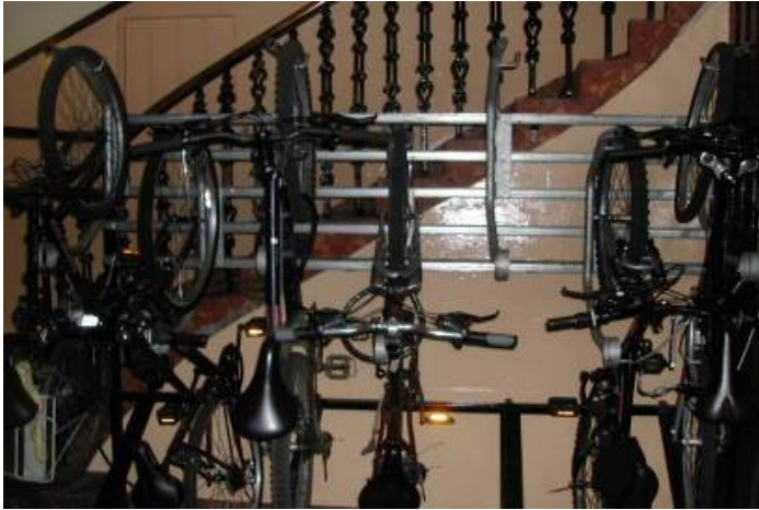
Stairwell vertical bike racks, bespoke [TPi]
