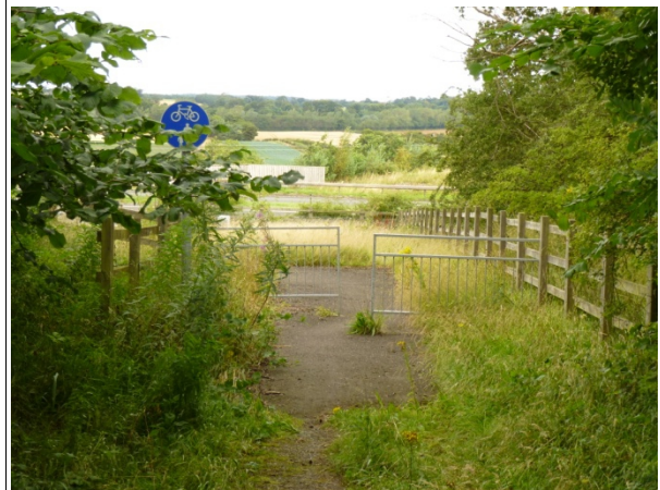
Approach to underpass
