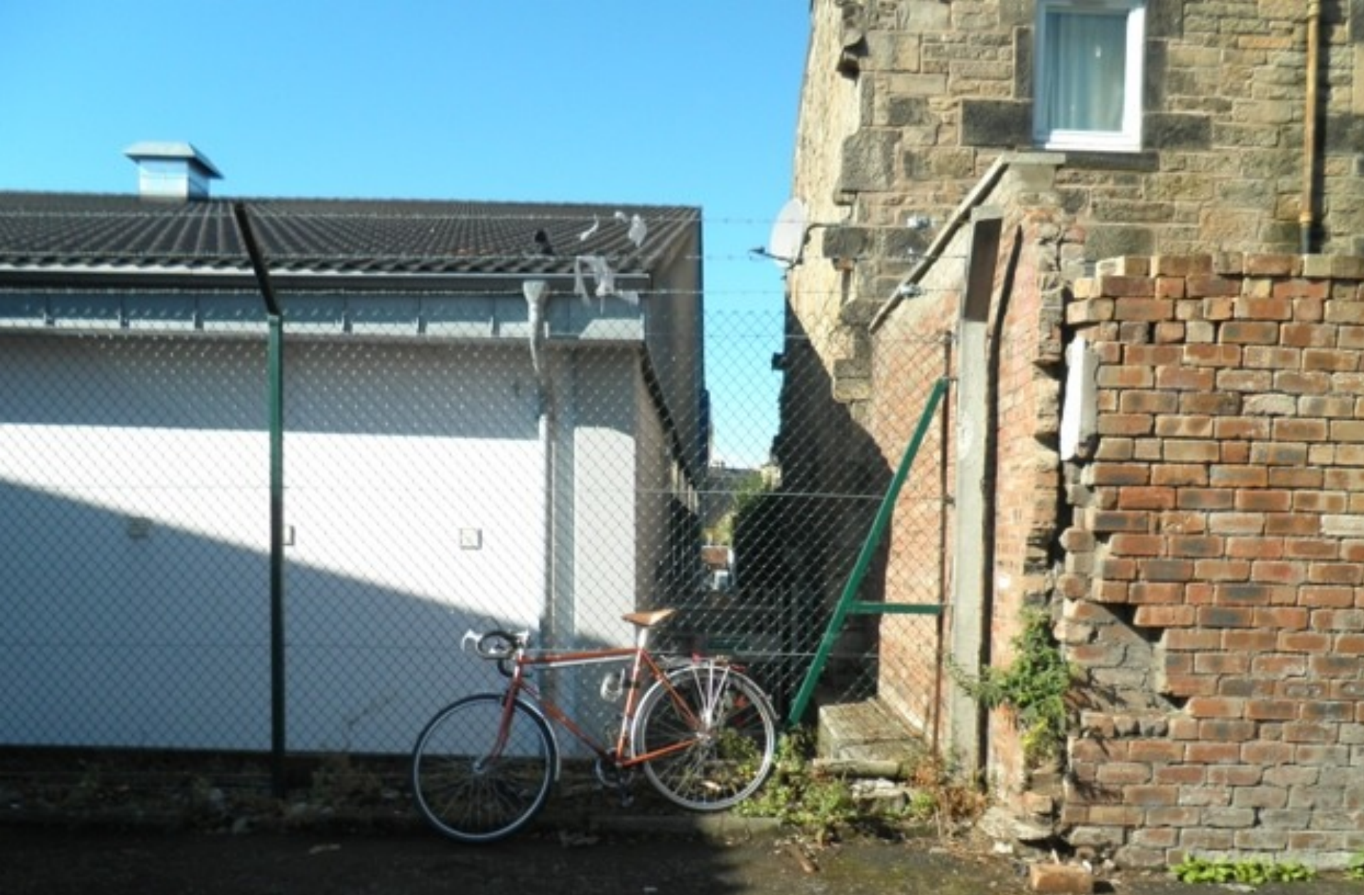
View of same gap, from opposite direction.
