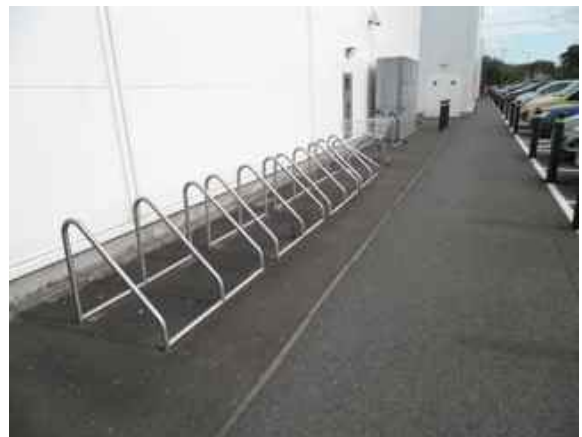
Tesco, C'phine 4: the official cycle park: racks (but with insufficient support), exposed, secure, remote (60 secs walk).
