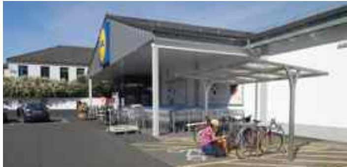
Lidl, Dalry Road - racks, under cover, secure, convenient - Rating: 1
