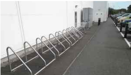
Tesco, Corstorphine official cycle park - racks with insufficient support, exposed, secure, remote (60 secs walk) - Rating: 4
