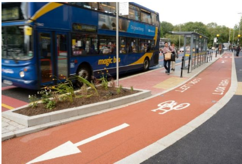
Figure 2.2: Photo of trial bus stop
