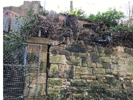
Figure 2 Displaced masonry
