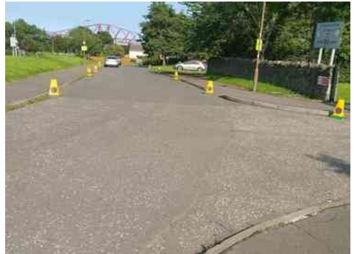
Service road, recommended for closure north from the school entrance
