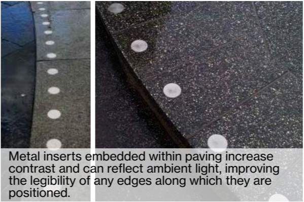
Photovoltaic in-ground marker lights are already in use along much of the canal towpath.
