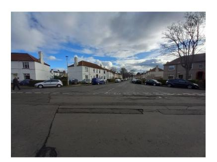
Photos showing a 'raised table' and a 'continuous footway', both of which improve the visual priority for people walking and wheeling across the side street junction
