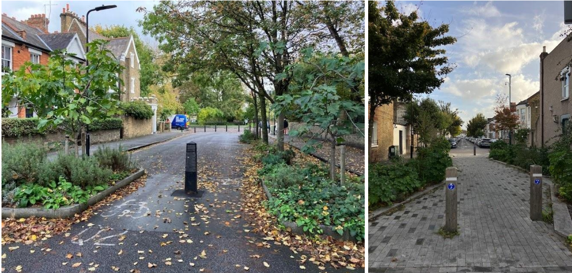
Examples of modal filters in the London Boroughs of Hackney & Waltham Forest.
