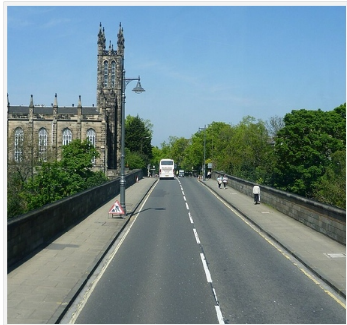
Cycling implication: If tram uses the Orchard Brae route, onroad cycling conditions will suffer, with the likelihood of more tramline injuries. Dean Bridge will be particularly problematic given its narrowness.
