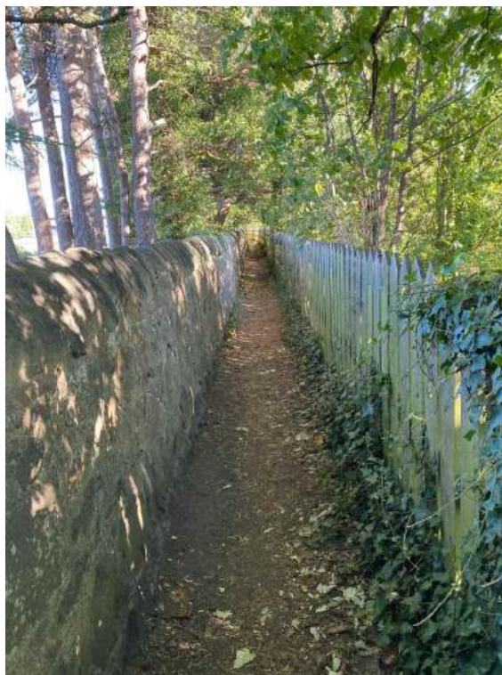
Fig 2: The existing poor quality walking path.
