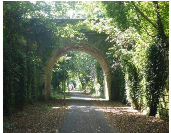
Approaching the tunnel on North Edinburgh path
