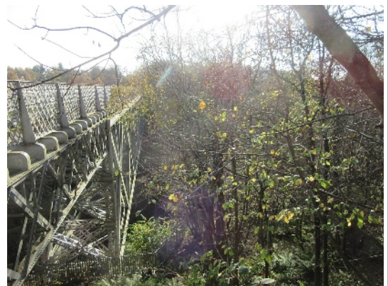
Bilston Glen viaduct
