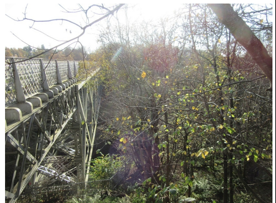
Bilston Glen viaduct
