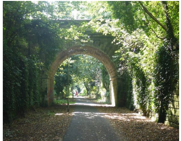
Approaching the tunnel on North Edinburgh path
