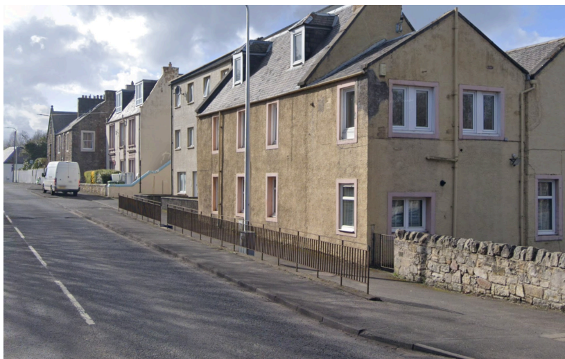
Existing guardrail proposed for retention at Westpans which will be a hazard for cycles - Google Streetview
