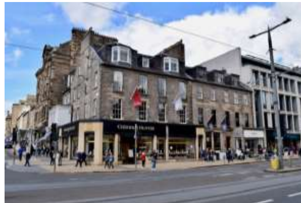
Above: An example of the original Georgian scale Princes Street buildings at 94-98 Princes Street.
