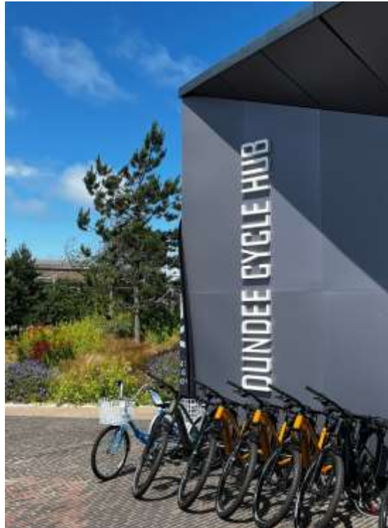
Dundee Cycle Hub, sited next to the V&A on the waterfront provides for servicing, retail, bike hire and a café, complementing the adjacent public realm.
