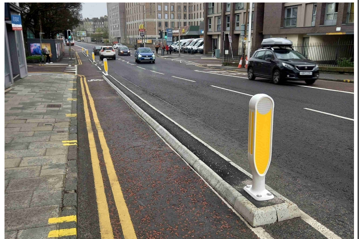
London Road bike lane installed during resurfacing
