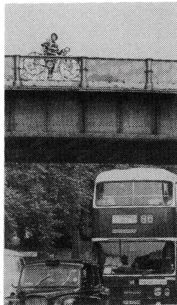
Cyclepath or another road? — The Roseburn railway bridge Photo: Chris Hill
