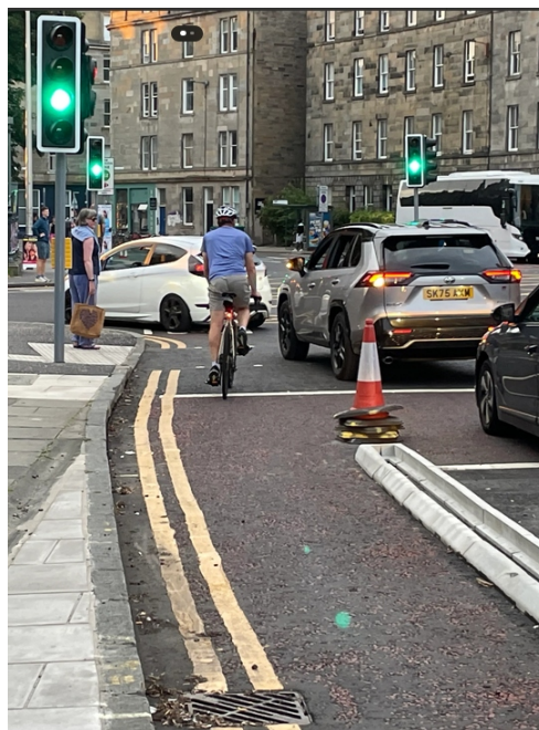
Summerhall resurfacing project (with changed bike lanes). A left-turn car lane allows cars to emerge as cyclists have green 'ahead' lights, producing a severe left-hook danger pic: Blackford Safe Routes
