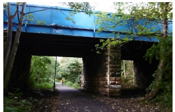
Newhaven Rd Overbridge Dave Attrill on flickr
