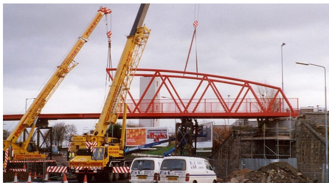
The Red Bridge is installed photo: Tim Smith
