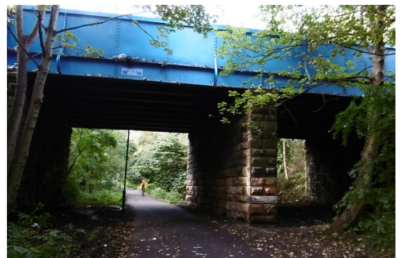
Newhaven Rd Overbridge Dave Attrill on flickr
